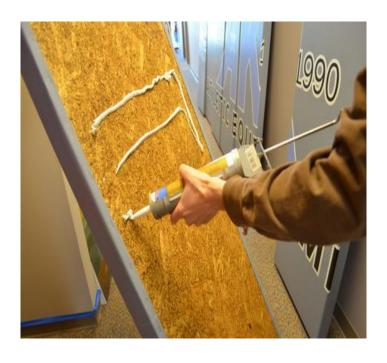
Before attaching wall pad, squeeze a small amount of liquid nails adhesive (found at most hardware stores) on the back middle portion of watch wall pad to ensure wall pads will stay firmly and evenly pressed against the wall.
