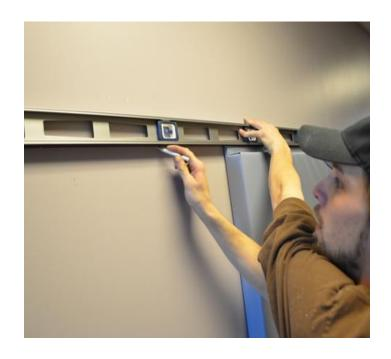
Each wall pad should be anchored into at least one stud, use a stud finder to find where your studs are located and make a small mark above your guideline for reference.
